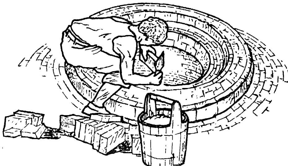
Fig. 4-12. Bricking the mouth of the pit without support.
