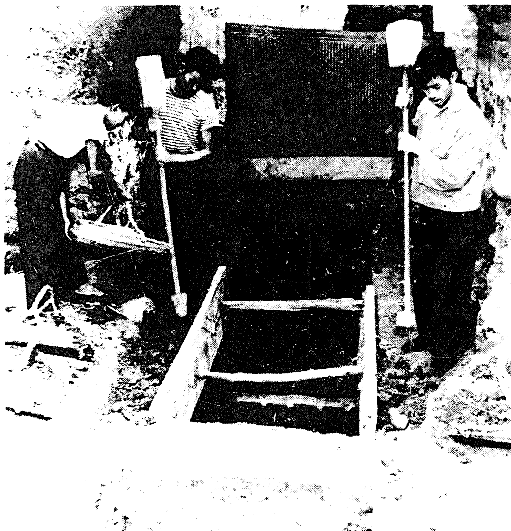
Plate 4-3. Pounding the walls firmly in making a rectangular pit of triple concrete.
