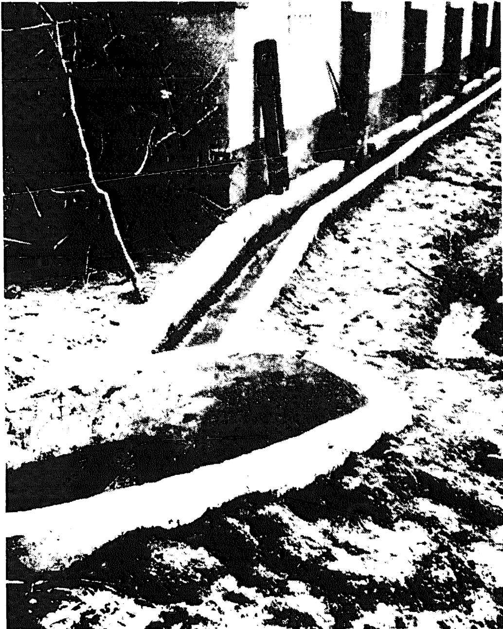
Plate 6-1. Piggery built with direct flow of animal wastes into biogas pit inlet.
