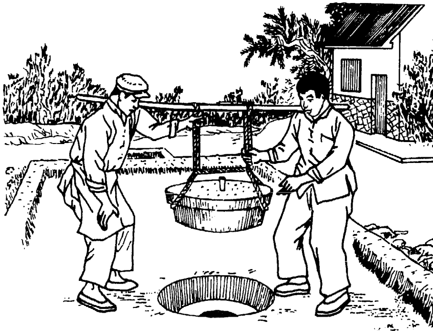
Fig. 4-23. Fitting a removable cover.
