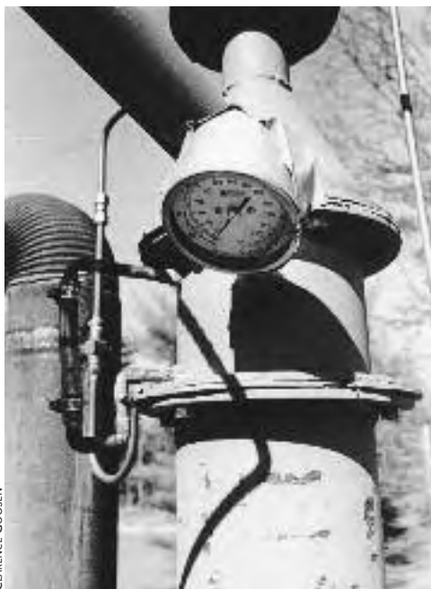
Fig. 8.7: An analog thermometer with probe is often the least costly option for temperature monitoring. If access is a problem, a remote thermistor with digital readout can be used.
