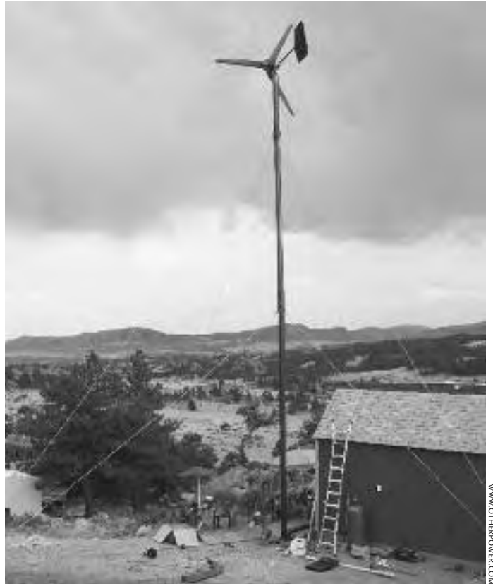
Fig. 7.12: At a good wind site, a homebuilt or commercial wind turbine can supplement heating requirements for a small ethanol fuel operation. New "homebrew" permanent magnet designs are very inexpensive on a per-watt basis.
