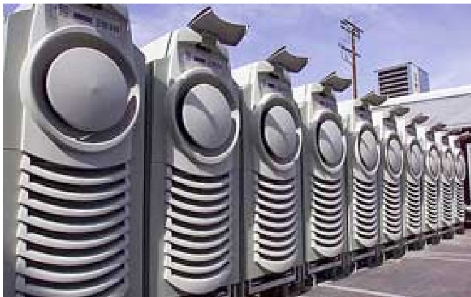
Gas Fired Microturbine
